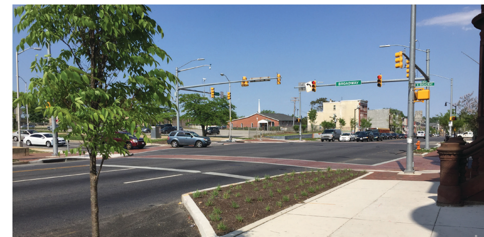
Recently completed E. North Avenue streetscape
